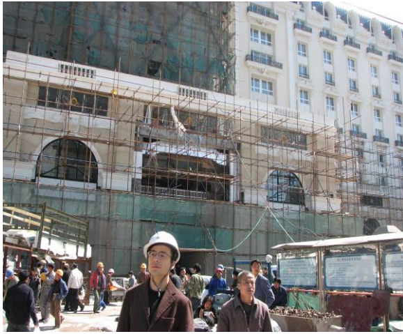
Darryl Agon on the Legendale construction site in 2008
